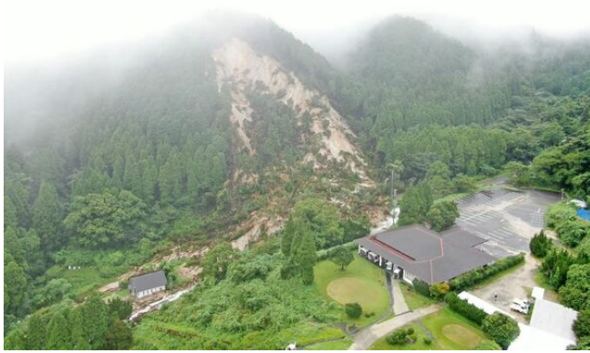
(b)Photo of Collapsed Area
