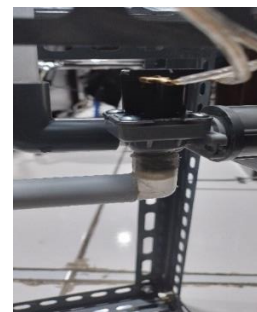
Fig. 14. Solenoid valve testing
