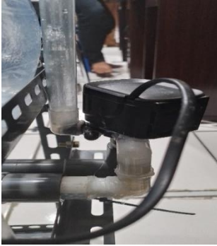
Fig. 15. Water pump testing
