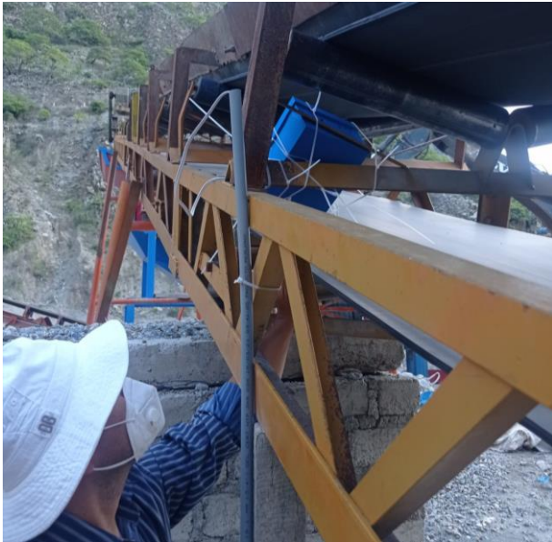
Fig. 9. Installing the prototype in the conveyor belt of ECONSA company.
