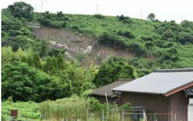
(a) Collapsed Area.
