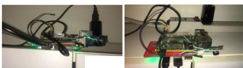
Fig. 6. Complete Hardware Setup during Runtime.
