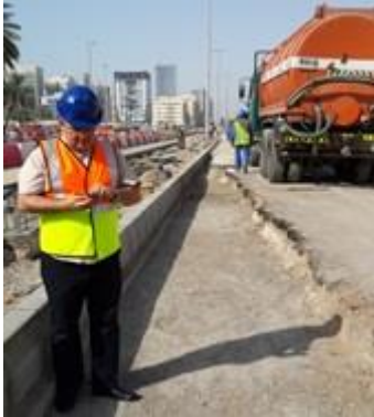
Fig. 6. Project Manager using MoSIC in Abu Dhabi
